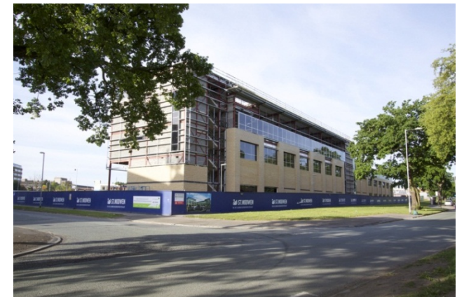
Etrop Court, Wythenshawe – 50,000 sq ft offices for Manchester City Council
